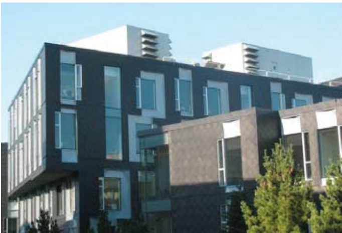
Gates Center with two of the roof mounted SEMCO systems.
