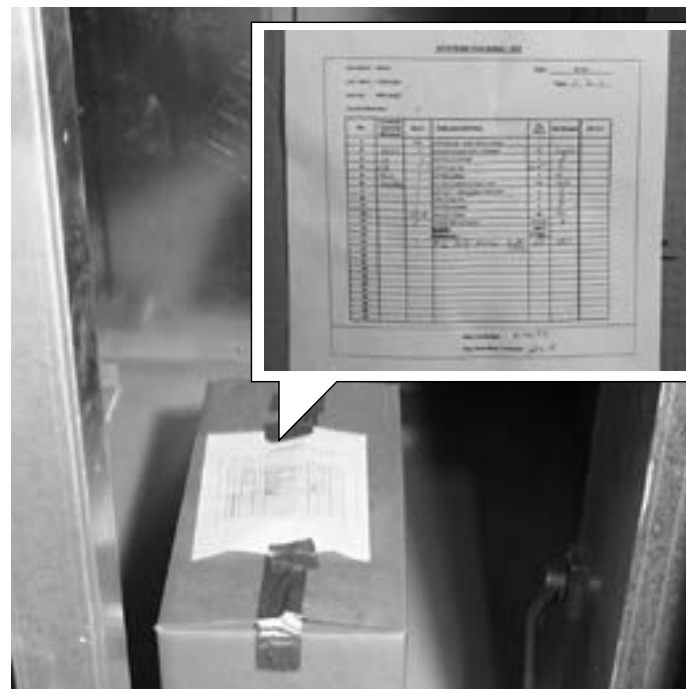
FIGURE 4. All gaskets, bolts, and other items required for installation are shipped in a box located in the supply air compartment. On top of the box you will find a packing list.
