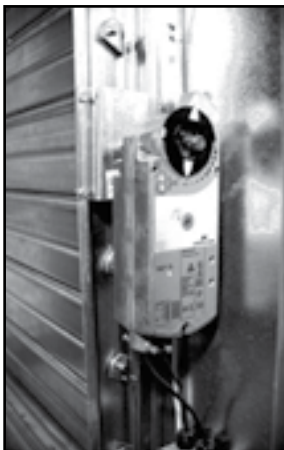
FIGURE 30. Damper actuator.
