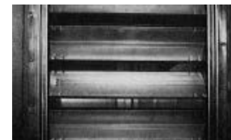
FIGURE 29. Be sure that damper blades open and close properly and have sufficient rotation clearance.
