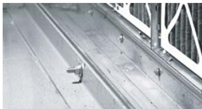
FIGURE 9. Field joint located at floor.
