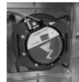
FIGURE 24 Wall mounted EC fan
