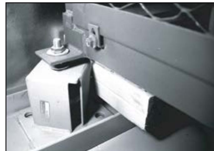
FIGURE 27. As an option, the fans can be mounted on seismic arrest mounts.
