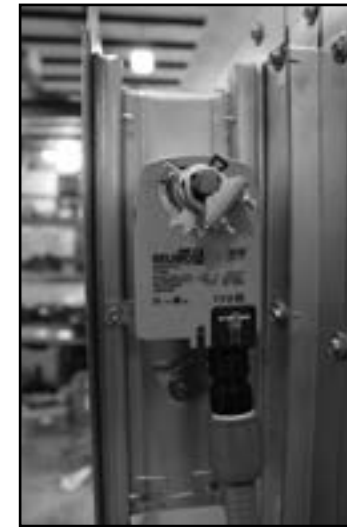
FIGURE 12. Damper actuator
