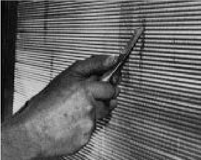
FIGURE 16. A fin comb may be used to remove matter entangled in fins, as well as to straighten fins. But normally flushing coils with water under normal pressure will remove most matter.
