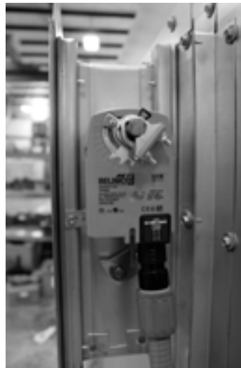
FIGURE 21. Damper actuator
