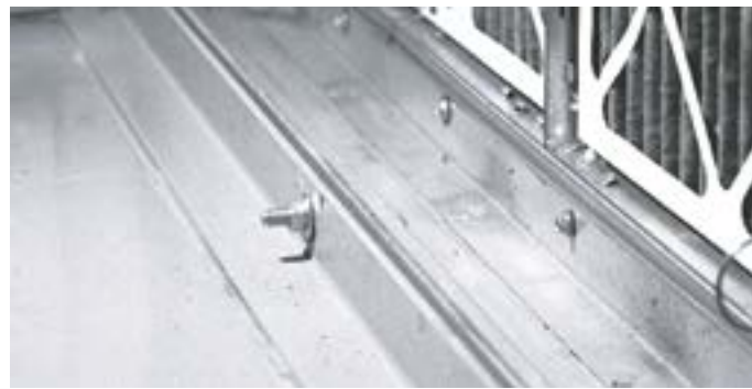
FIGURE 7. Field joint located at floor.
