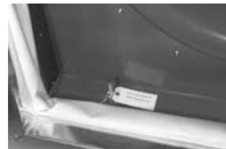
FIGURE 16. Two restraints in the fan inlet which bolt the fan to the base rail.
