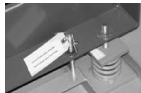
FIGURE 17. Two restraints at the base of the rear of the fan.
