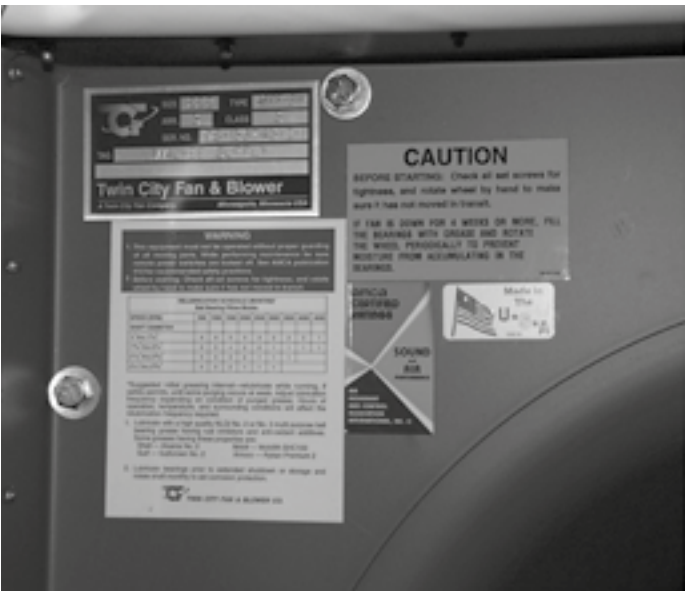
FIGURE 23. The lubrication label for larger fans is located on the fan inlet housing.*Fan model/brand may vary based on the project.
