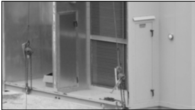
FIGURE 1 Lift modules only with lugs located at the base of each module. Do not use a forklift. NOTE: Chain hoists used to level unit.
