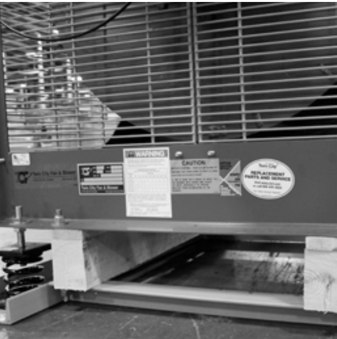
FIGURE 22. All fans installed in FläktGroup SEMCO systems are labeled with lubrication instructions that should be followed. On smaller fans the label can be found on the fan frame. *Fan model/brand may vary based on the project.
