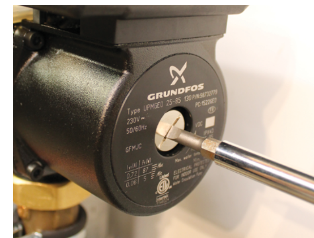
FIGURE 7 If the pump air locks, manually rotate the center cap on the pump to vent.
