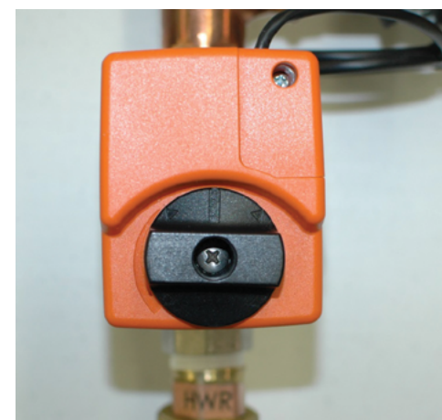
FIGURE 5. Actuator control valve with the dial shown in closed/bypass mode. Press and rotate 90 degrees for open mode.
