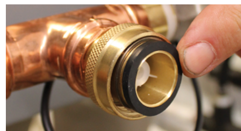
FIGURE 4. Place provided o-rings on all pipe connections.
