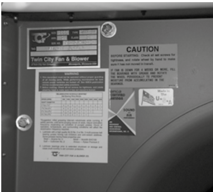
FIGURE 34. The lubrication label for larger fans is located on the fan inlet housing.
