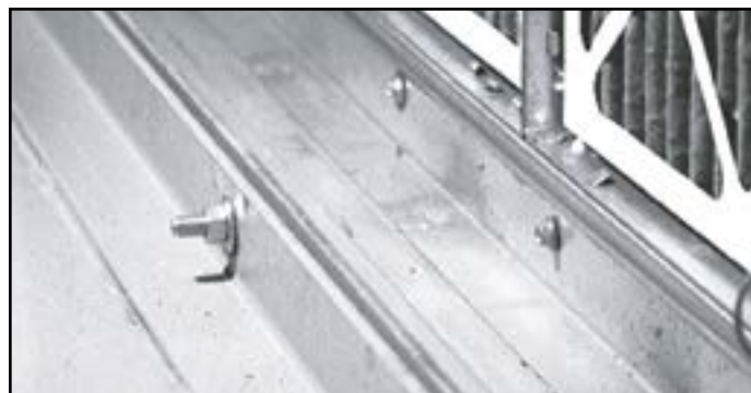
FIGURE 7. Field joint located at floor.
