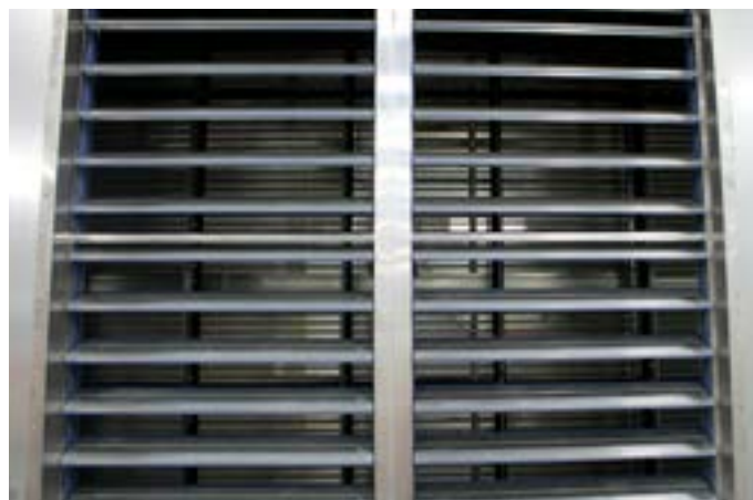
FIGURE 27. Be sure that damper blades open and close properly and have sufficient rotation clearance.
