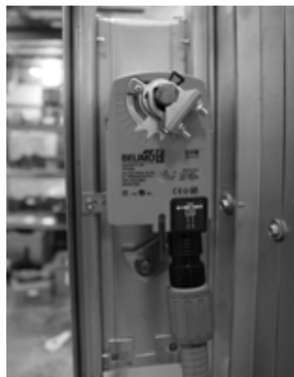
FIGURE 28. Damper actuator.
