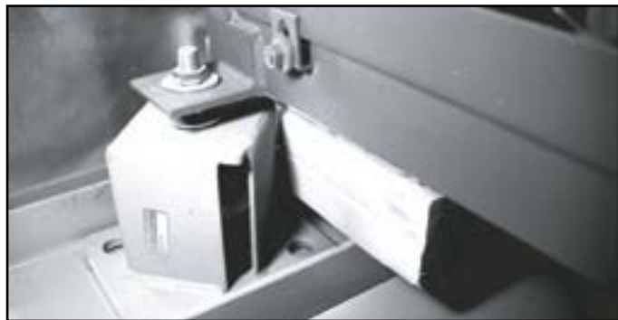
FIGURE 26. The fans may be mounted on seismic arrest mounts NOT STANDARD
