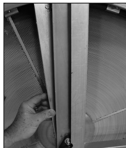
FIGURE 43. Sheet Metal Frame purge section removal.
