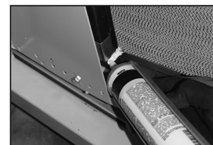
FIGURE 29. Caulk purge seal where it meets perimeter seal.
