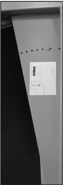
FIGURE 36. The purge section on the wheel.
