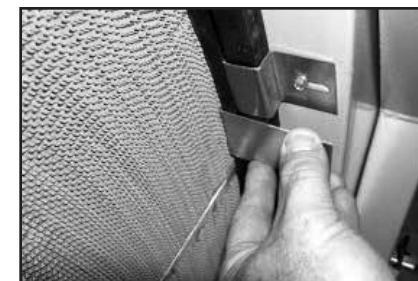
FIGURE 26. Loosen clip and insert gauge. Adjust seal to correct gauge depth.
