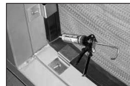
FIGURE 30. On the weather side of the wheel caulk where face seal meets perimeter seal at both ends.
