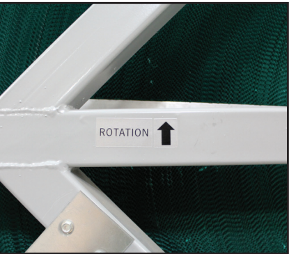
FIGURE 16. Don't let ductwork hide rotation or airflow arrows.
