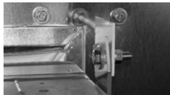
FIGURE 21. Two restraints at the top of the fan bolting the fan to the fan wall.
