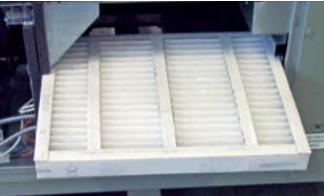
FIGURE 14. Replacing return air filters.
