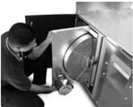
FIGURE 33. The wheel cassette is removable through the service door.
