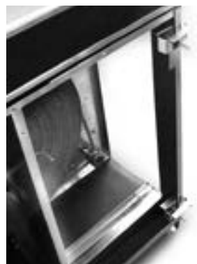
FIGURE 18. View of brackets installed.
