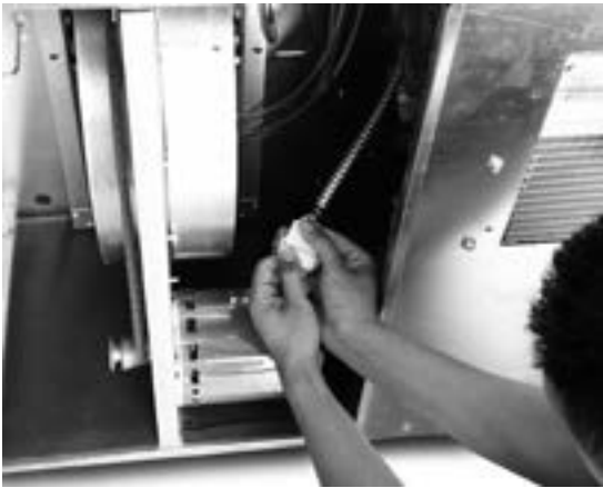
FIGURE 31. Prior to sliding out the wheel cassette, the wheel motor quick release must be disconnected.
